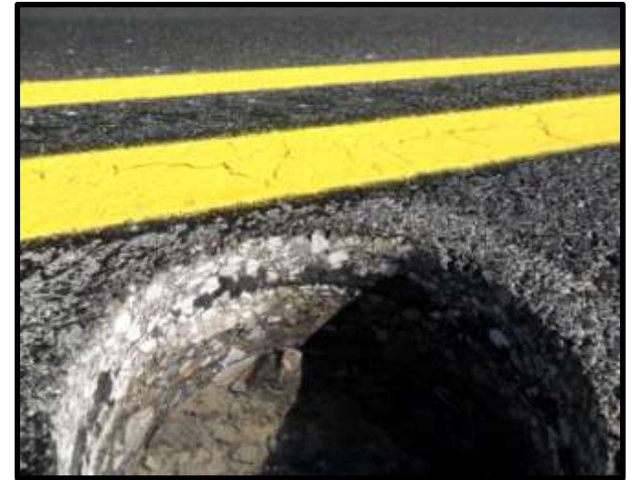
Notched Wedge Joint Core Hole
