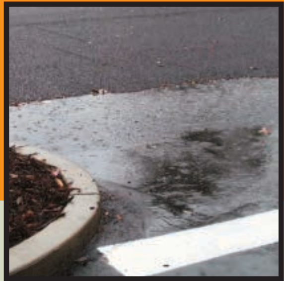
Figure 1 – As seen in this photograph, rainfall runs off traditional impervious asphalt but drains through the porous asphalt parking spaces.
