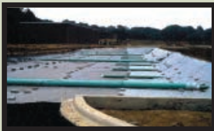
Figure 5 – Perforated pipes distribute stormwater evenly throughout the infiltration bed. Geotextile allows water to drain but prevents soil movement into stone.
