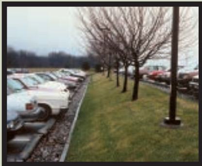
Figure 3 – Porous pavement parking bays are “benched” down a hillside.
