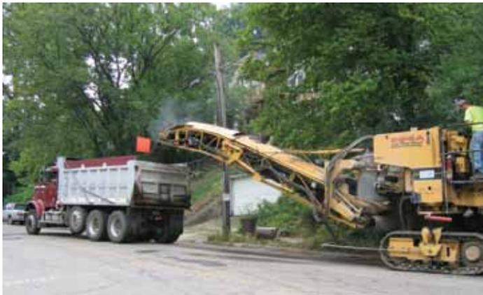
*Milling machine reclaims RAP from a deteriorated surface.*
