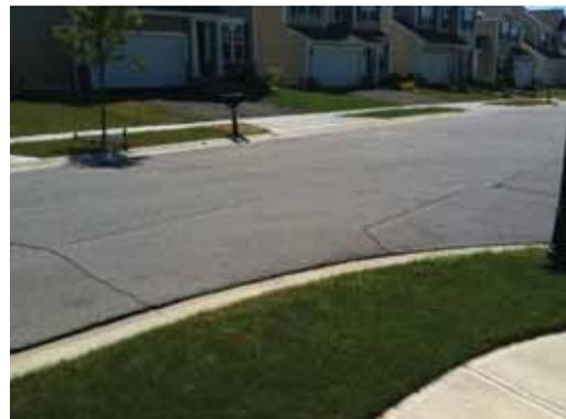
*Reflection cracking is occurring on an asphalt surface atop a concrete base.*
