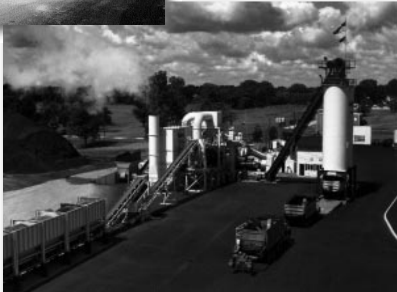
Mar-Zane Plant 21 AFTER
