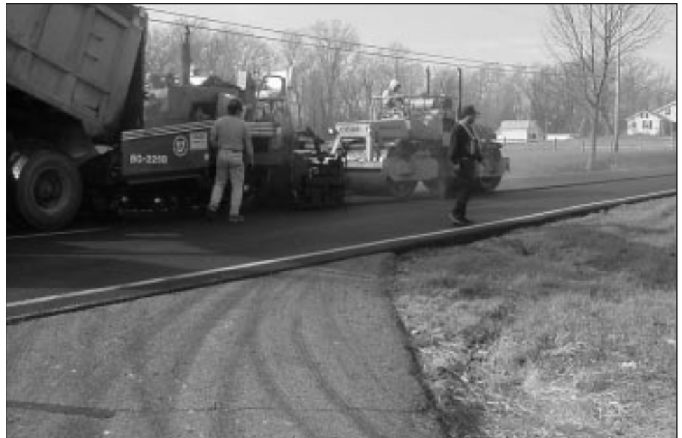
SR 422, Geauga County, Schloss Paving Company crew placing polymer/fiber mix.
