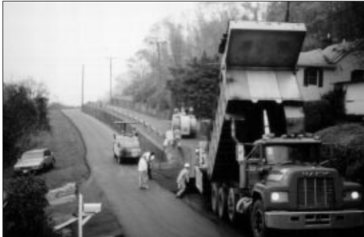
Tri-State Asphalt Company resurfaces County Road 24 with 1 1/2 inch surface course.
