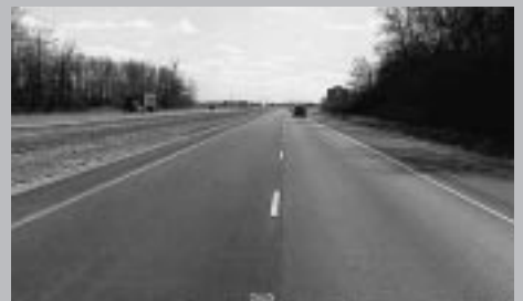
Interstate Route 280 From the Ohio Turnpike to Lemoyne Road, Wood County Project 504 (199)
