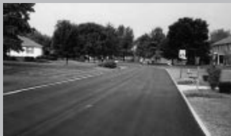
Vienna Park Resurfacing Project Montgomery County, Ohio
