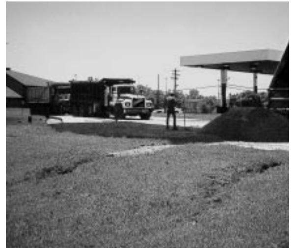
The damaged pavement was replaced with 12 inches of aggregate base, and 6 inches of bituminous aggregate base, prior to a finishing 2 inch overlay.
