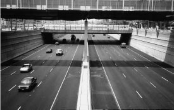
Fort Washington Way Stone Mastic Asphalt (SMA) surface placed.
