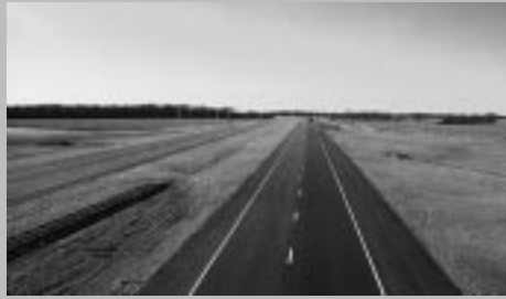
Construction of U.S. Route 35 in Greene County, near Jamestown, Project 259 (1998)
