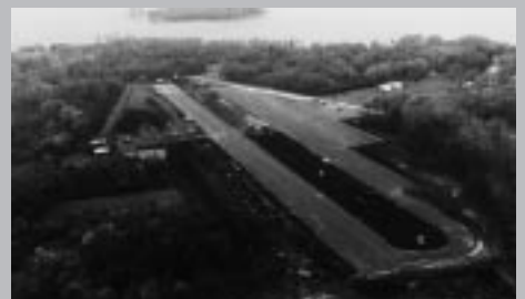
Middle Bass Island Construction of Runway 10-28 Put-In-Bay Township Port Authority
