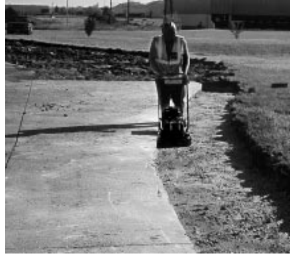
The damaged pavement was replaced with 12 inches of aggregate base, and 6 inches of bituminous aggregate base, prior to a finishing 2 inch overlay.
