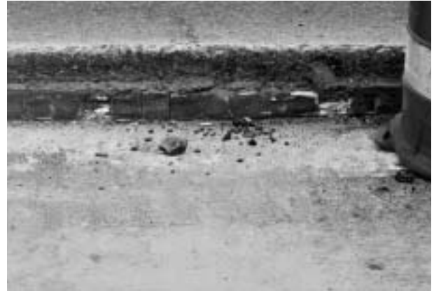
Removal of the asphalt surface and bricks leaves room for 8 inches of new, rut-resistant asphalt.
