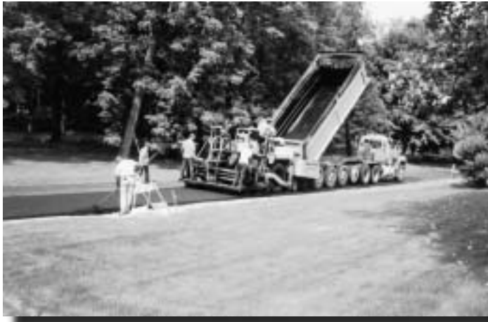
Wagner Paving crew doing what they do best.
