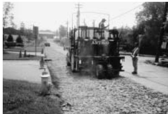
Rubblization of the concrete pavement proceeded rapidly.
