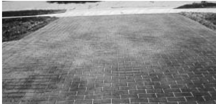
New asphalt driveway finished in simulated brick pattern.
