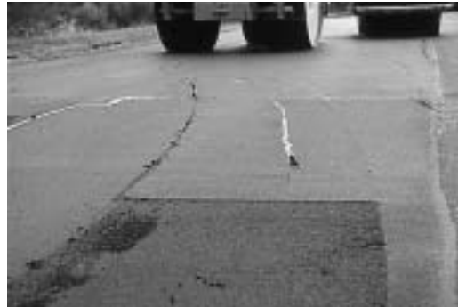
Placing Type B mixture on SR 261 near Kent (1994)
