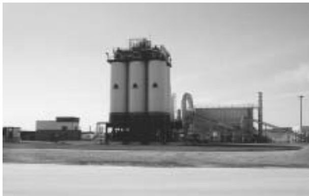
Kokosing Materials, Inc. Columbus Plant in Columbus, Ohio
