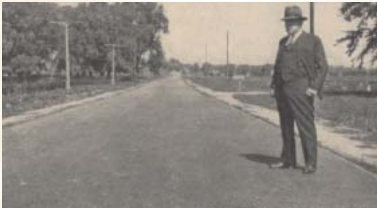
Clifford W. Simpson inspects and approves U.S. Route 27 after it has been re-surfaced with asphalt
