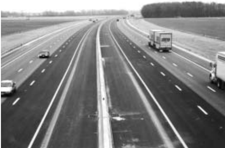
This finished pavement constructed near milepost 89 by the S.E. Johnson Company, Maumee, Ohio allows greater mobility for the 44,000+ vehicles per day that traverse Northern Ohio on the Ohio Turnpike
