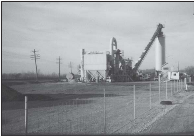
Cisle Asphalt Plant, Augsberger Road, New Miami, Ohio
