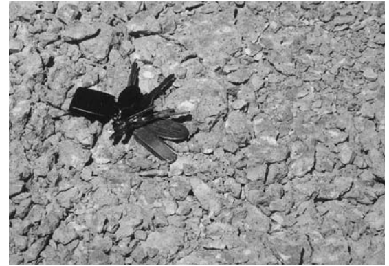
Rubblized concrete pavement on Medina 271.
