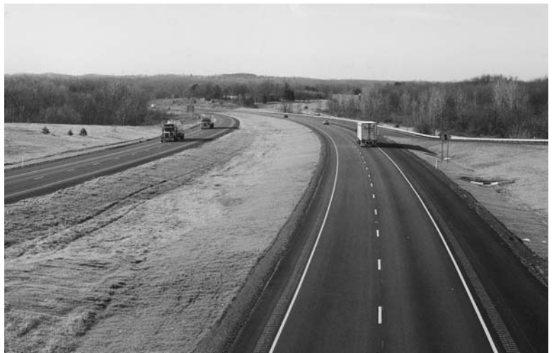
Pavement rehabilitation on Medina 271 completed.
