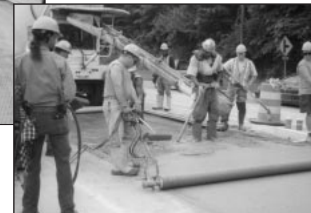
UTW being placed.
