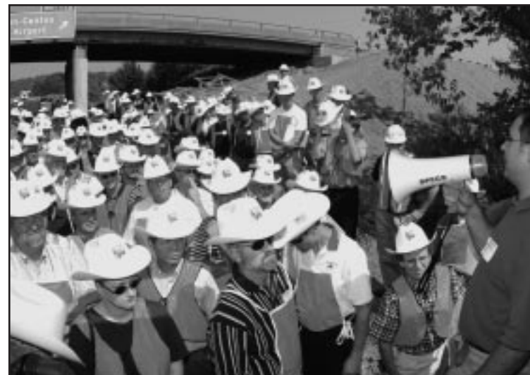
Open house attendees visit I-77 construction site to view work in progress.
