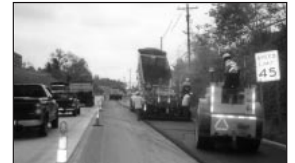
Type 1H surface, PG 76-22M, hard as rocks.
