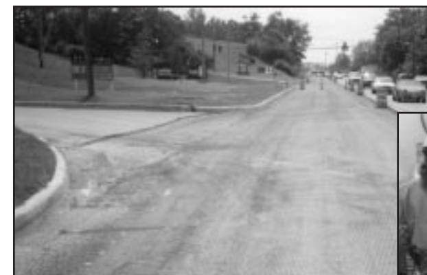
Harrison Pike milled for placement of the ultra-thin whitetopping (UTW).
