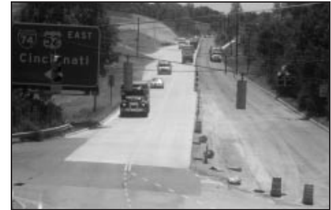
UTW open to traffic, up-grade lanes being milled for asphalt resurfacing.
