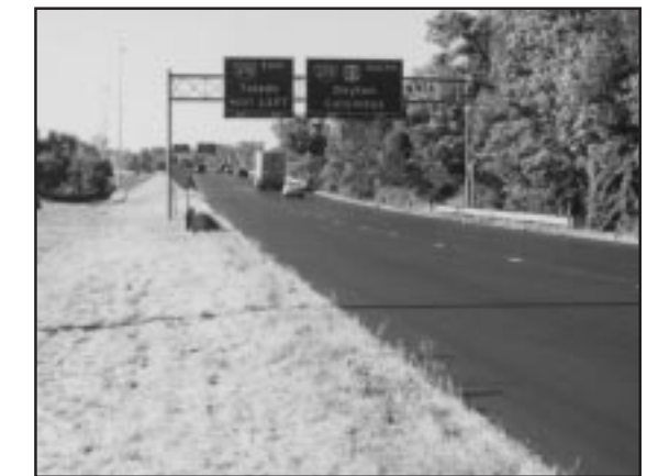
Nighttime paving keeps traffic moving on US23. Smoothseal placed this September.
