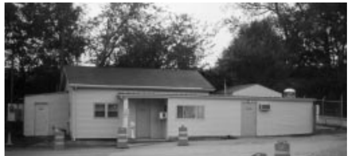
Remodeled office at Barrett's Carthage facility.
