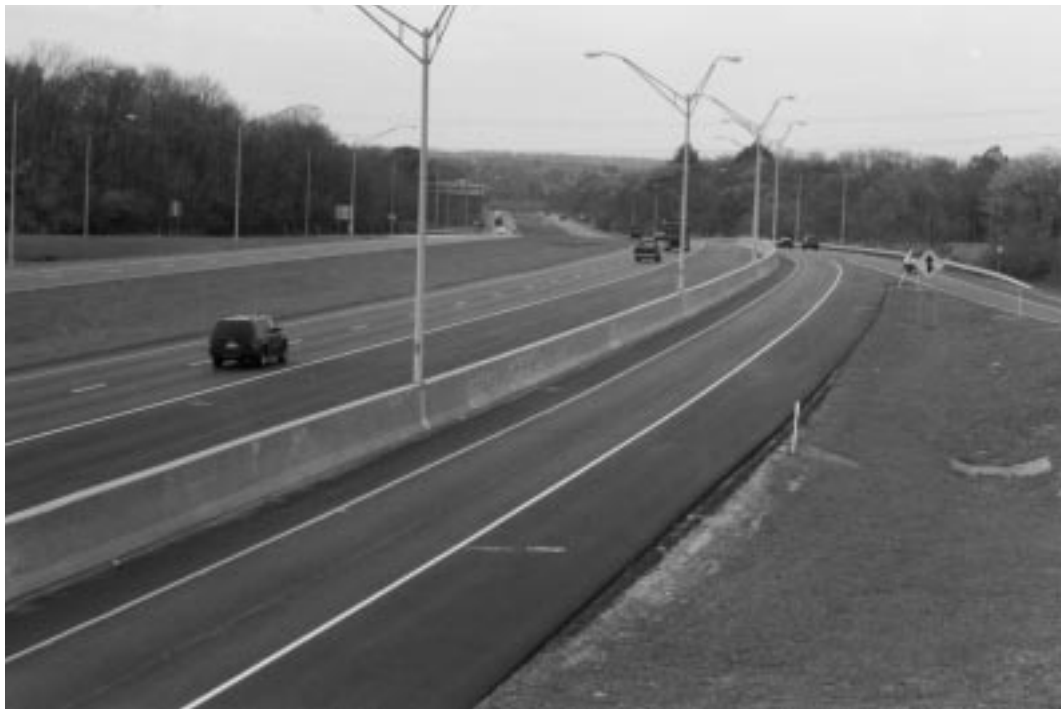
High Quality Superpave placed on I-74.
