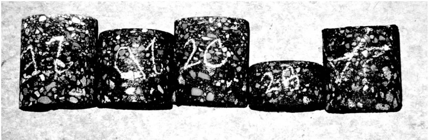
Fig. 2 Cores taken from an overlay on a brick pavement show 2 1/2 inches of rutting in a nominal 4 1/2-inch-thick, three-course overlay. All three asphalt layers were deformed, with the greatest deformation in the bottom, Type 2, layer.
