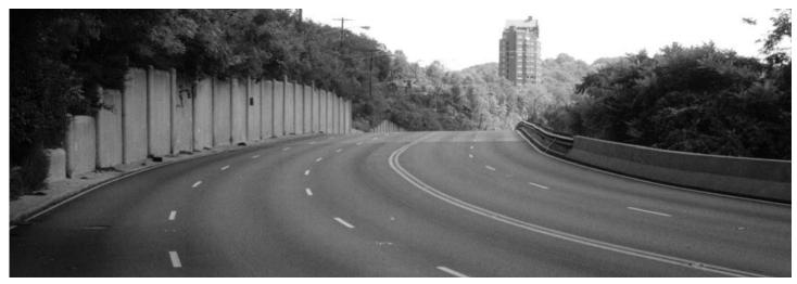
Cincinnati's Columbia Parkway provides motorists a quiet ride, better visibility during the night because of less headlight glare, and less chance of hydroplaning during wet conditions because of the use of OGFC.
