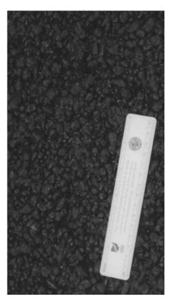
(above) Open-Graded Friction Course, such as this used on Columbia Parkway in Cincinnati, features course aggregate that is bound by a heavy coating of polymer-modified asphalt.
