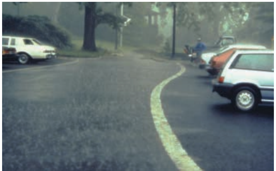
This photograph of the parking lot at Philadelphia's Morris Arboretum, taken during Hurricane Floyd, shows how stormwater will pool on the conventional driving surface and be absorbed through the porous pavement in the parking bays.
