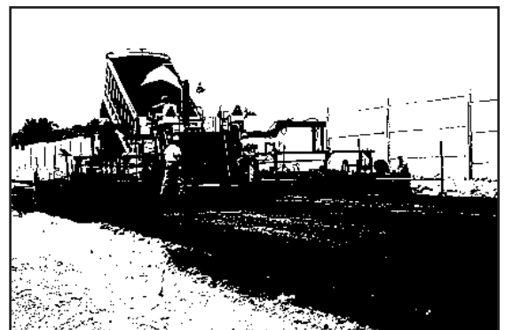
Kokosing experiments with paving full width of 38 feet with their modified paver.
