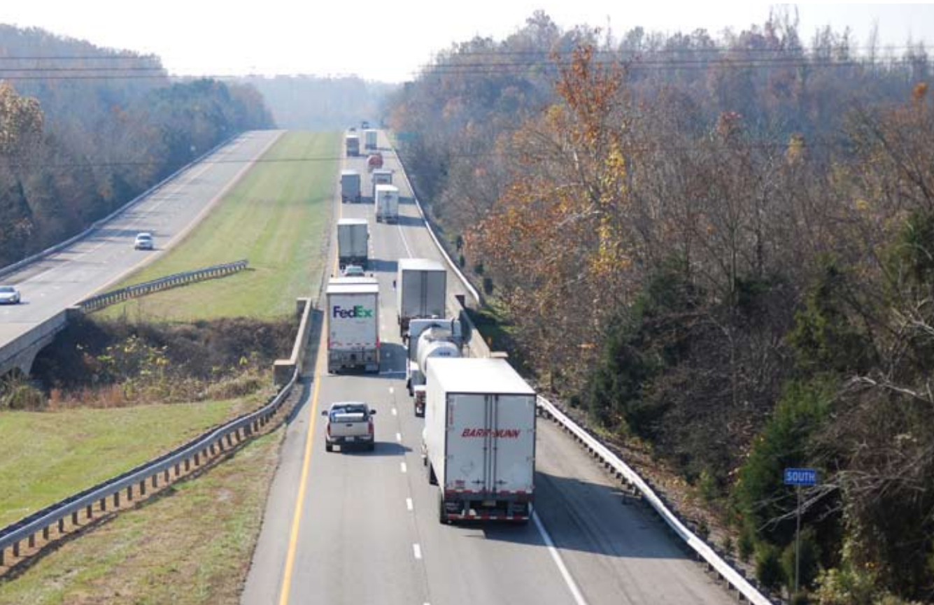
The Arkansas State Highway and Transportation Department received a 2009 Perpetual Pavement Award for Highway 134-North, Miller County, US 71, Section 2.
