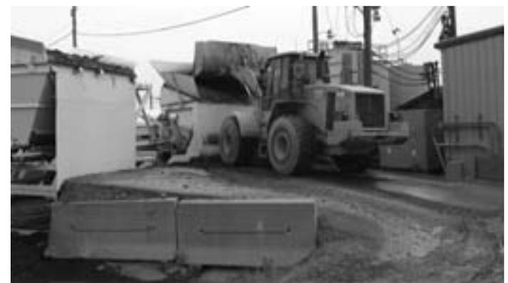
*RAP from the stockpile is loaded across a coarse screen into the RAP cold-feed bin.*
