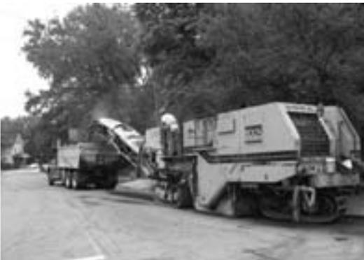
**The reclaiming of asphalt pavement begins with the milling of an existing road surface. It is estimated that Ohio contractors reclaim 2.6-million tons of asphalt pavement per year.**
