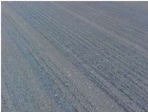
Figure 5 – Non-uniform tack-coat application (photo courtesy of the Ohio Department of Transportation)
