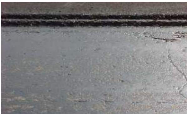
Figure 1 –Uniform tack-coat application (photo courtesy of the Ohio Department of Transportation)
