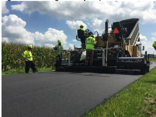
Figure 1: Paving Thinlay Asphalt.
