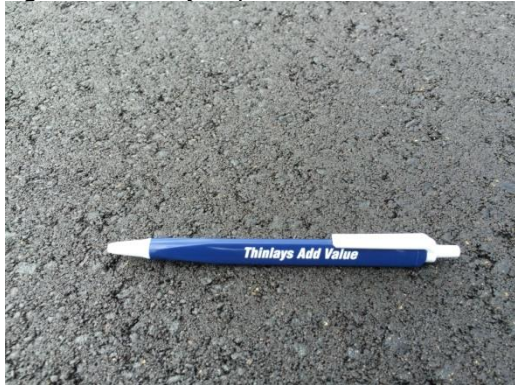
Figure 2: Thinlay Asphalt Concrete mat texture.
